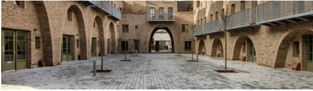
McGrath Road by Peter Barber Architects © Morley von Sternberg
