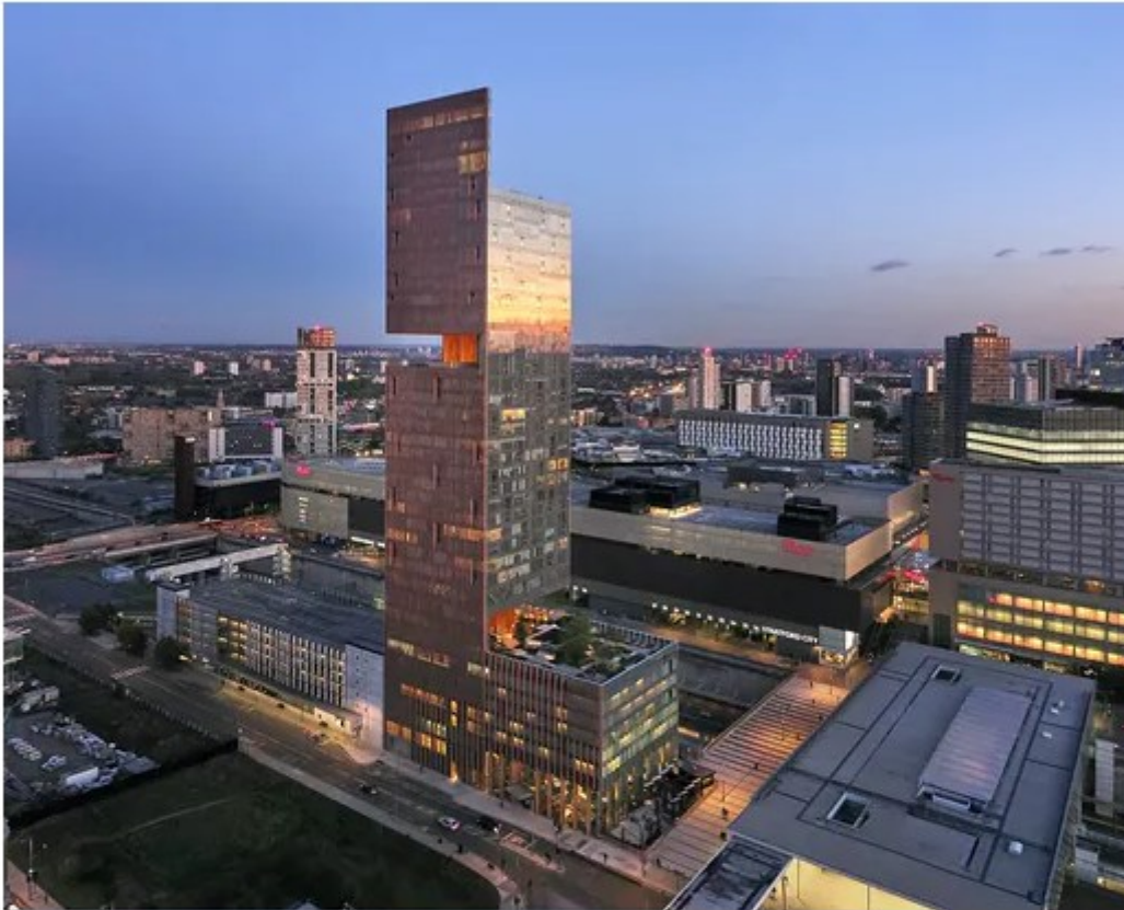
Manhattan Loft Gardens by Skidmore, Owings & Merrill © Hufton - Crow
