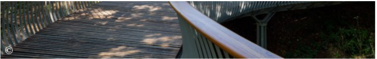
Tintagel Castle Footbridge for English Heritage (Cornwall) / Ney & Partners and William Matthews Associates
